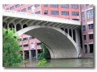
San Jacinto Street Bridge is an open spandrel concrete arch bridge, sister to the Montgomery Viaduct, or the Main Street Bridge. This
