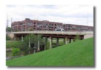
Sabine Street Bridge is a cantilever concrete span bridge. It replaced the old iron and wood Heiner Street Bridge.
